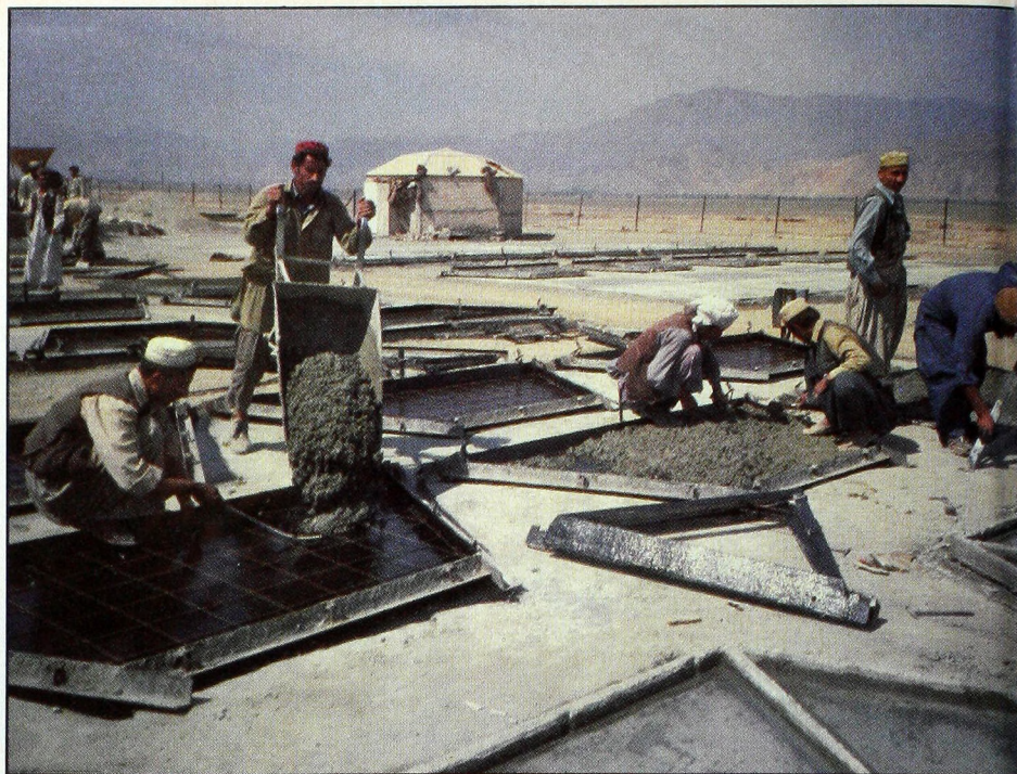
Concrete geodesic dome construction provides durable shelter—and jobs—for refugees.
