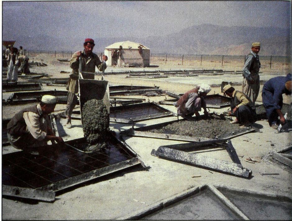
Concrete geodesic dome construction provides durable shelter—and jobs—for refugees.
